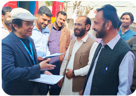
The visit of Mr. Doc - Construction Manager UNICEF to monitor the minor repair & maintenance work.
